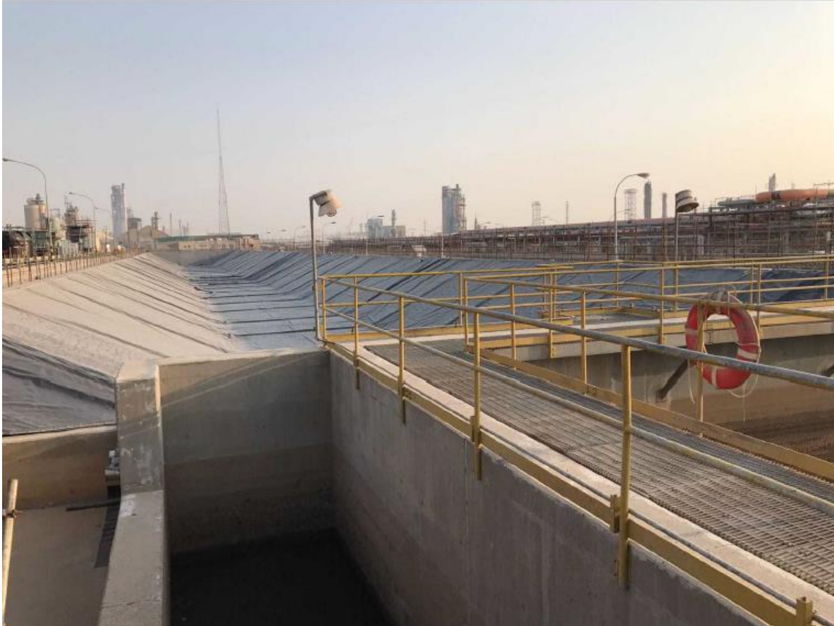
Figure 9 : Geo Membrane- Completely installed in the basin
